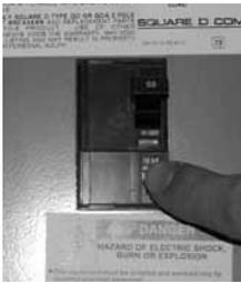
*\*The Swim Spa GFCI breaker or disconnect should be located in a weather proof box close to the spa, but no closer than 5 feet. This applies to the Crosstrainer 2 and Crosstrainer SJ only. The H2X and Crosstrainer have this breaker mount behind smoked plastic doors on the front panel.*
