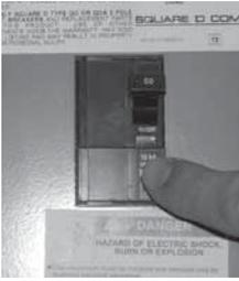
*\*The Swim Spa GFCI breaker or disconnect should be located in a weather proof box close to the spa, but no closer than 5 feet. This applies to the Crosstrainer 2 and Crosstrainer SJ only. The H2X, Crosstrainer and Momentum have this breaker mount behind smoked plastic doors on the front panel.*
