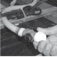
1. **DRAINING YOUR LEGACY SPA.** The drain is located behind the front panel on the far right side, grasp the hose bib cap and turn it counter clockwise. Attach a garden hose, if desired. Turn the black knob on the side of the valve a quarter turn. Draining times may vary by model using the external hose bib. A sump pump may also be used to drain the spa quickly.
