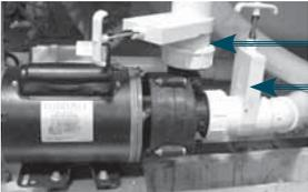
Turn on power to the swim spa. If your spa is equipped with two electrical supplies, make sure that they are both turned on. The swim spa will go through its priming mode. This lasts approximately 5 minutes. The purpose of the priming mode is to help insure that the jet pumps have been primed with water and are ready to operate. It may be necessary in some instances to bleed air from the jet pumps
