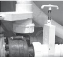
Be sure all pump and heater unions are secure. Each pump has 2 unions and the heater has 2 unions. A newly delivered swim spa may have loose unions caused in transporting the swim spa. Check that all slice valves are open, in the up position. Again, the slice valves may become closed during transportation of the swim spa.
