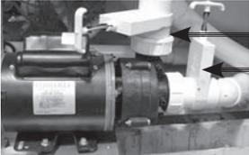
Turn on power to the swim spa. If your spa is equipped with two electrical supplies, make sure that they are both turned on. The swim spa will go through its priming mode. This lasts approximately 5 minutes. The purpose of the priming mode is to help insure that the jet pumps have been primed with water and are ready to operate. It may be necessary in some instances to bleed air from the jet pumps
