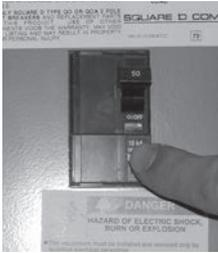
*\*The swim spa GFCI breaker or disconnect should be located in a weather proof box close to the spa, but no closer then 5 feet.*
