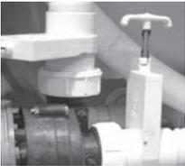
Be sure all pump and heater unions are secure. Each pump has 2 unions and the heater has 2 unions. A newly delivered swim spa may have loose unions caused in transporting the swim spa. Check that all slice valves are open, in the up position. The slice valves may become closed during transportation of the swim spa.
