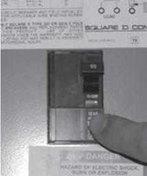
A ground fault circuit interrupter (GFCI) is required by the National Electrical Code for your protection. The tripping of the GFCI may be caused by a component on the spa or by an electrical problem. Electrical problems include but are not limited to, a faulty GFCI breaker, spa component, power fluctuations, or improper wiring. It may be necessary to contact an electrician if your dealer recommends doing so.
