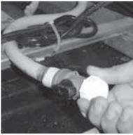
1. **DRAINING YOUR SPA.** The drain is located behind the front panel of the spa, grasp the hose bib cap and turn it counter clockwise. Attach a garden hose, if desired. Turn the black knob on the side of the valve a quarter turn. Draining times may vary by model using the external hose bib. A sump pump may also be used to drain the spa quickly. Be sure to replace the cap once the spa has been drained.
