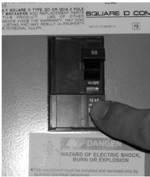
*The swim spa GFCI breaker or disconnect should be located in a weather proof box close to the spa, but no closer than 5 feet.*
