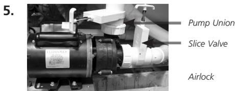
Turn on power to the swim spa. If your swim spa is equipped with two electrical supplies, make sure that they are both turned on. The swim spa will go through its priming mode. This lasts approximately 5 minutes. The purpose of the priming mode is to help insure that the jet pumps have been primed with
