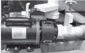
Turn on power to the swim spa. If your spa is equipped with two electrical supplies, make sure that they are both turned on. The swim spa will go through its priming mode. This lasts approximately 5 minutes. The purpose of the priming mode is to help insure that the jet pumps have been primed with water and are ready to operate. It may be necessary in some
