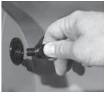
The Momentum 80 has an additional air bleed system that helps aid in relieving air locks. There is an air bleed valve located in the filter area of the swim spa portion of the swim spa. When filling the swim spa this should be opened to facilitate relieving any air that may be trapped in the pumps. Make sure that the plug is reinstalled once the spa is running correctly.
