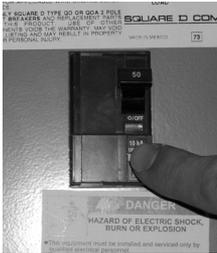
*The swim spa GFCI breaker or disconnect should be located in a weather proof box close to the spa.*
